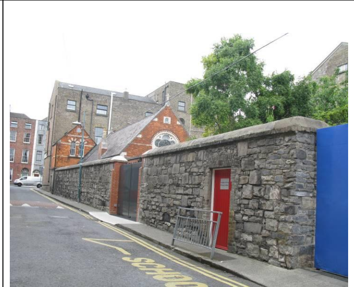
Rear site with Victorian chapel and entrances to National School
