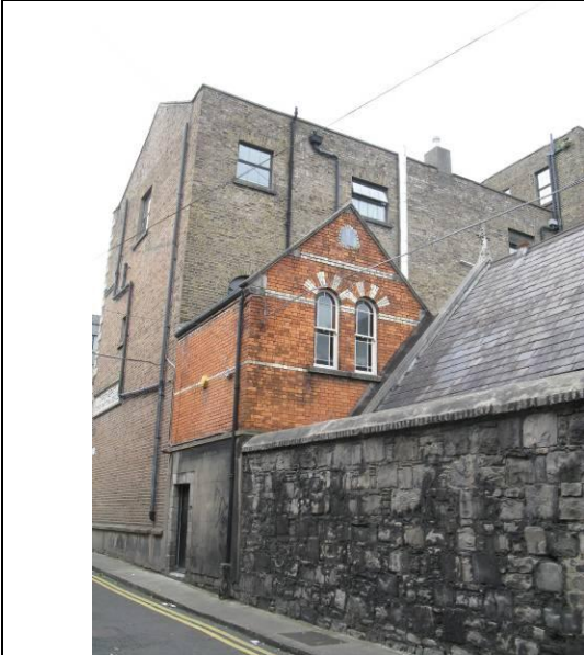
Rear elevation and Victorian return
