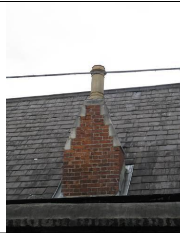
Chimney detail & natural slate roof to chapel
