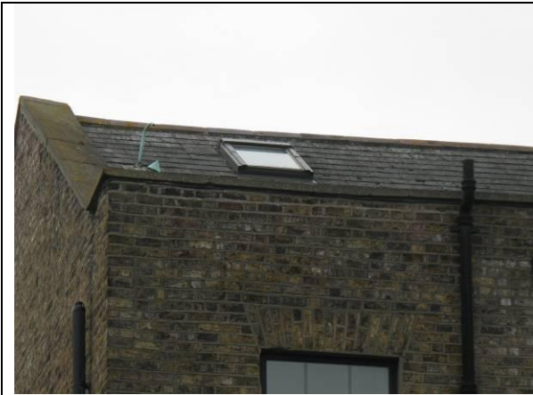
Attic storey to main convent
