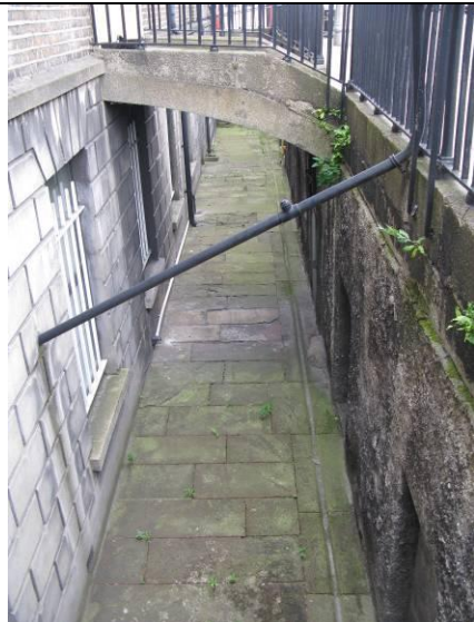
Front basement area
