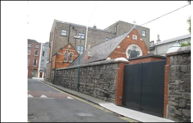
Rear elevation of convent with chapel and rear entrance
