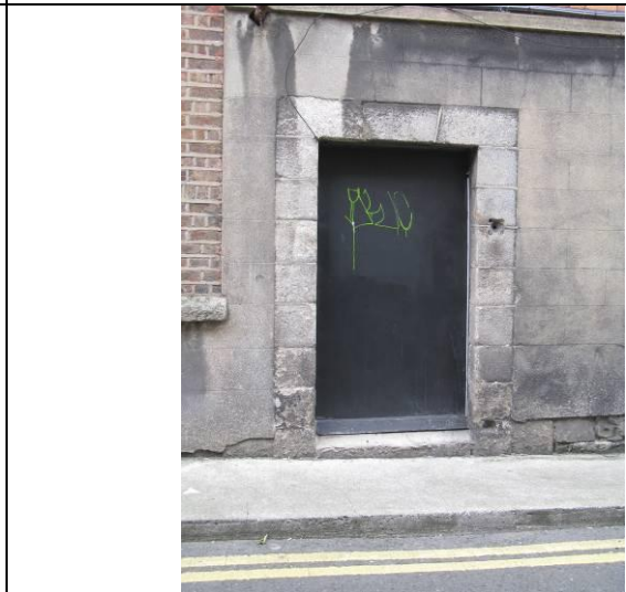
Pedestrian entrance with granite surround
